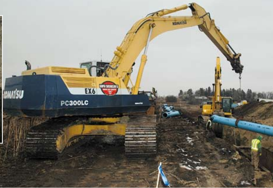
A Kemper Construction operator uses a Komatsu PC300LC-5 to lower 18-inch water line for the city of Minot. "It has a lot of power," Kemper Superintendent Rod Houle said of the excavator. "We don't have any problems with it and it's really good for lowering pipe down in the hole."
