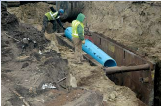
A Kemper Construction operator uses a Komatsu PC300LC-5 to lower 18-inch water line for the city of Minot. "It has a lot of power," Kemper Superintendent Rod Houle said of the excavator. "We don't have any problems with it and it's really good for lowering pipe down in the hole."
