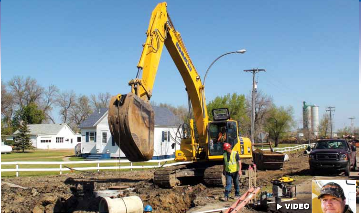
Operator Jamie Burnside (in cab and inset photo) places concrete pipe using a Komatsu PC360LC-10 on the West Fargo Main Avenue project. It's one of two Tier 4 Interim machines Sellin Brothers purchased in the past year. "They've proven to be just as good as any piece of Komatsu equipment we've ever had," said President Mark Sellin.
