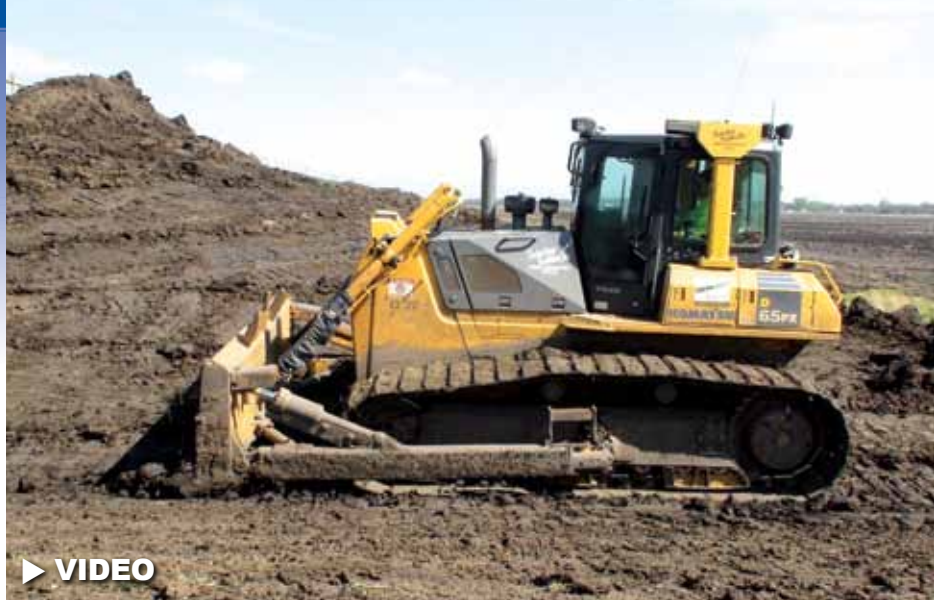
An Industrial Builders operator uses a Komatsu D65PX dozer to grade dirt at Fargo’s water-treatment facility.
