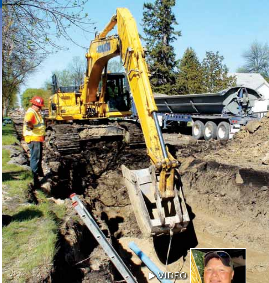
Operator Darwin Klemetson lowers pipe into a ditch with a Komatsu PC390 as part of a street reconstruction project in Warren, Minnesota. “It has good power and stability,” Klemetson said. “I like the rearview camera and the operator comfort. It’s a nice-riding machine.”
